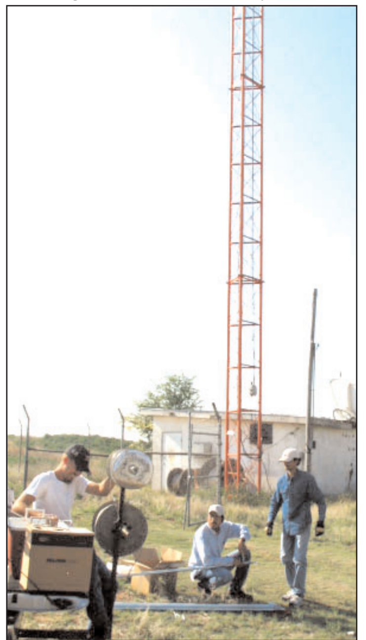
AEI crew preparing to install wind data equipment.
