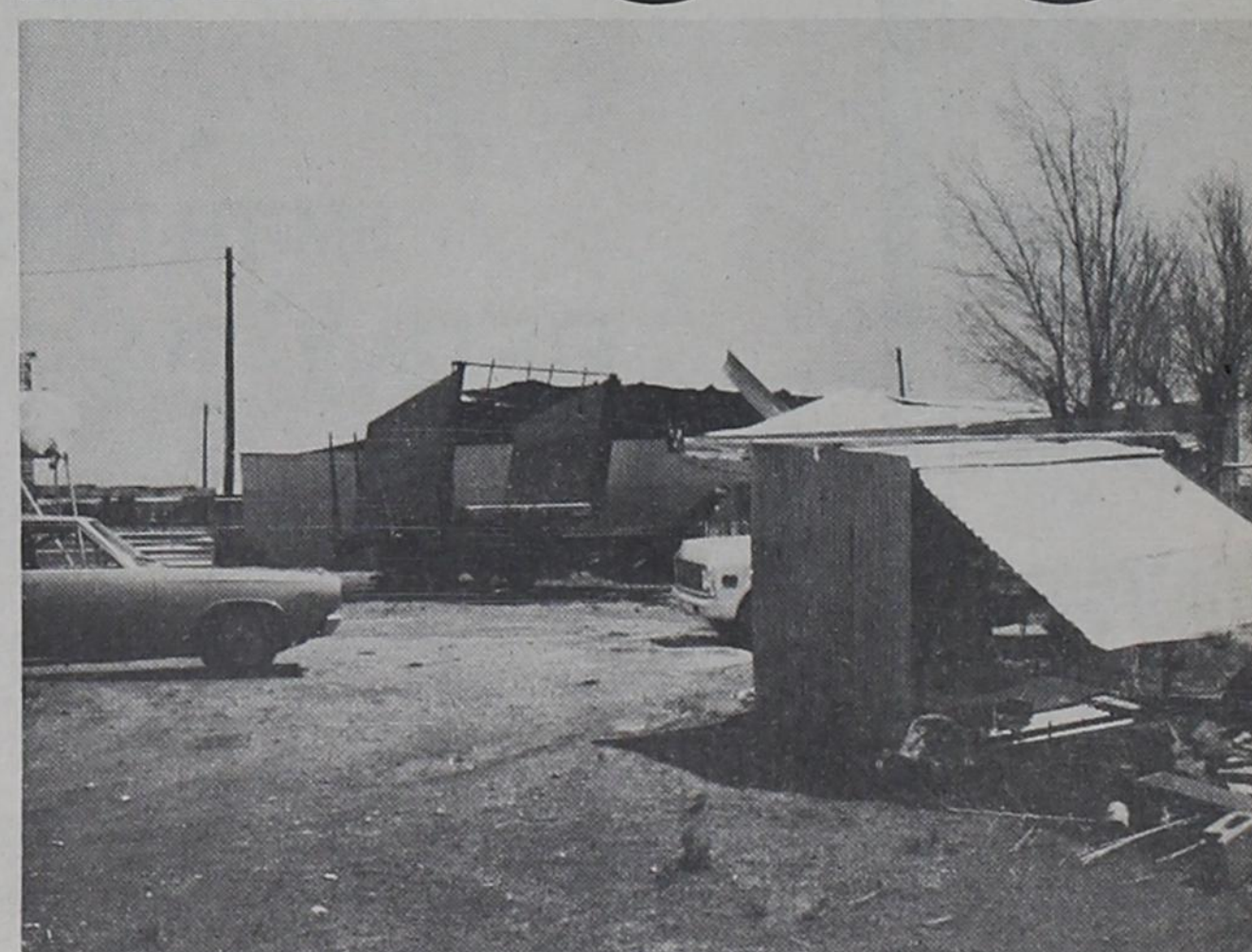
TWISTER TAKES ROOF - A small twister during Monday's spring storm lifted the roof from the barn and damaged the pump house on the Ben Mesman place in the Oklahoma Lane Community. High winds, dust, rain and hail were reported over the area, during the storm. Heavy pea-sized hail and .10 inch rain fell, but no crop damage was reported.
