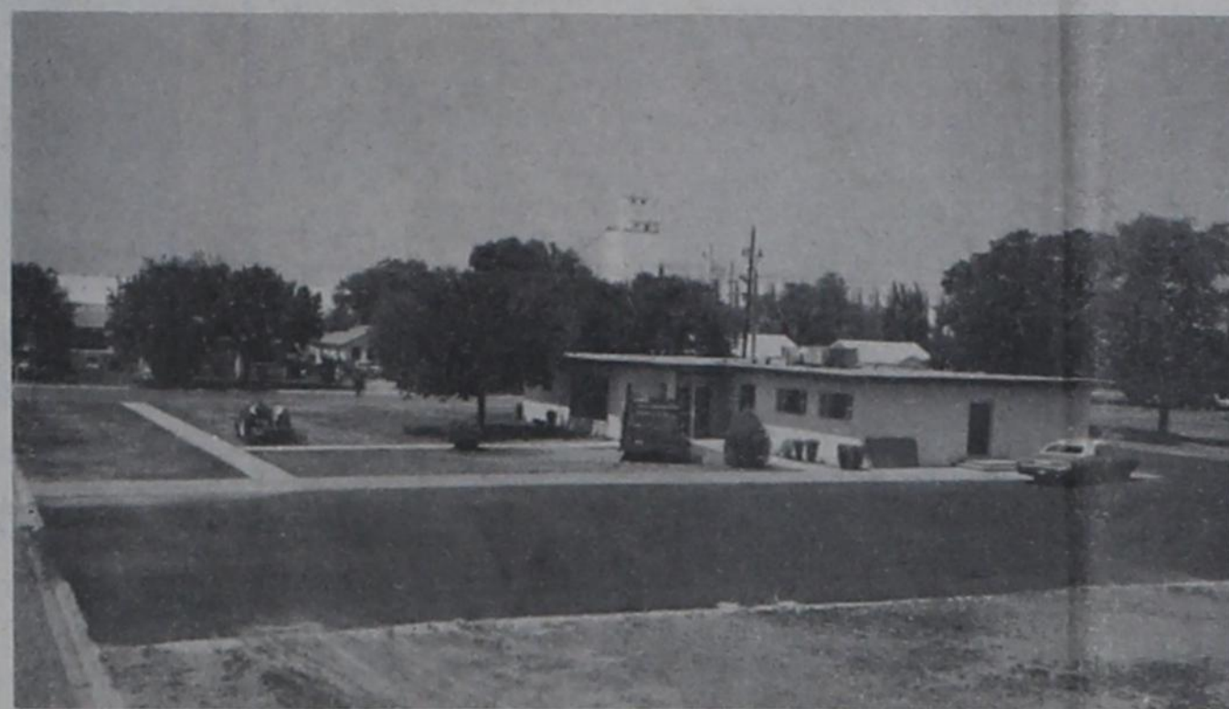
Work Nearing Completion
