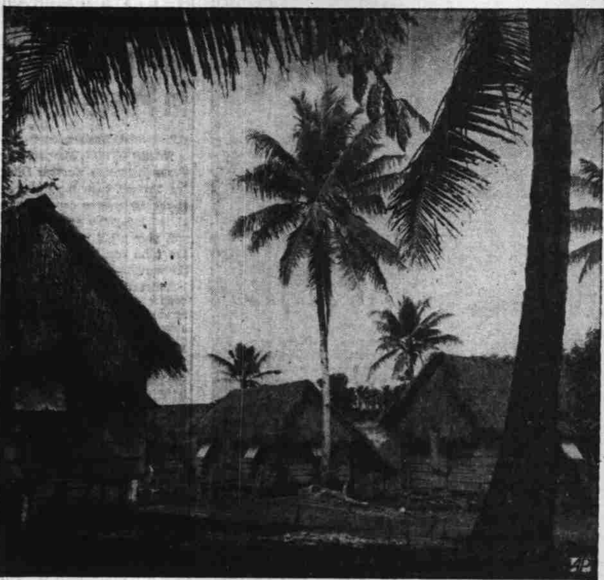
PACIFIC HOUSING PROJECT—Thatch-roofed homes built by U. S. civil affairs authorities provide shelter for natives whose homes were wrecked in battle.
