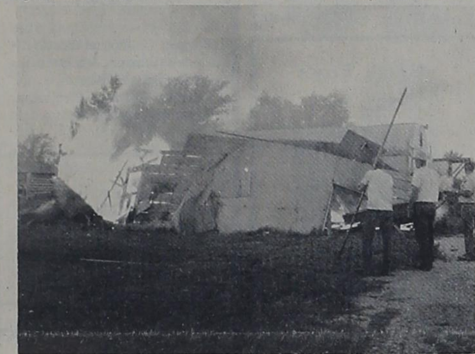
ALERT -- Texico volunteer firemen remained on the alert for some time Wednesday evening as they watched to see that a fire, which had been purposely set to destroy an old house which was in a state of collapse on Wheeler Ave., did not spread to adjoining property. Firemen found this a good way to get in some practice and at the same time improve the looks of the town.
