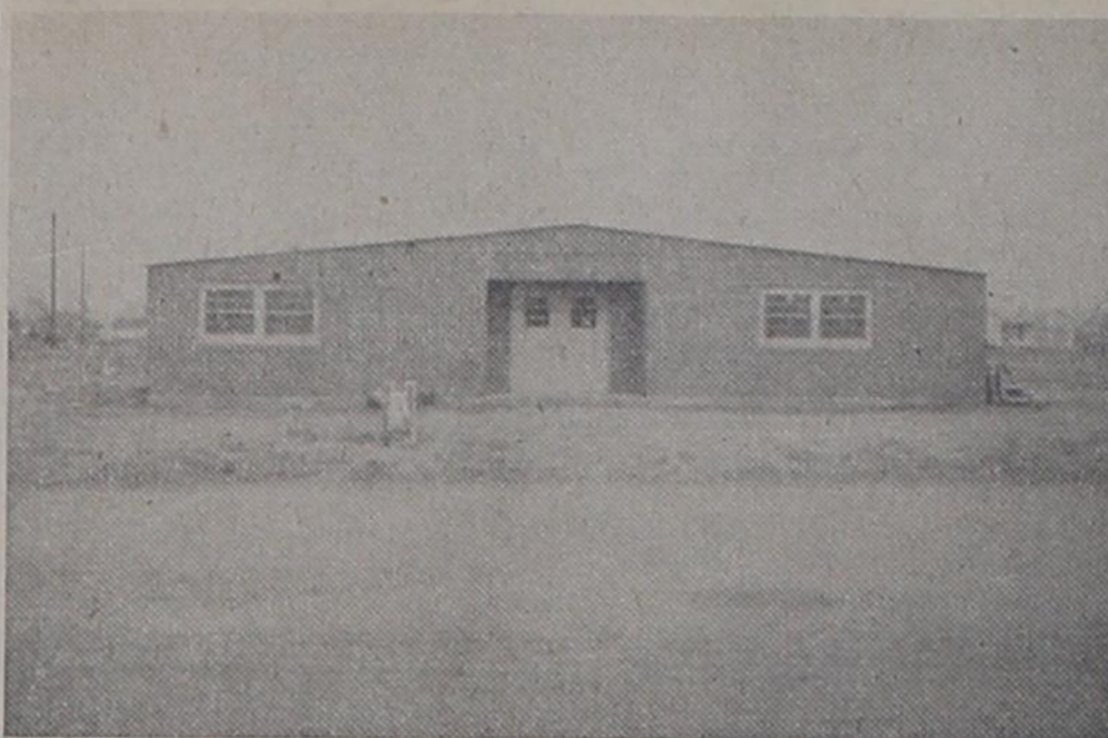
Pictured is the new home economics building for Bovina Schools, which has already been made ready for classes.
