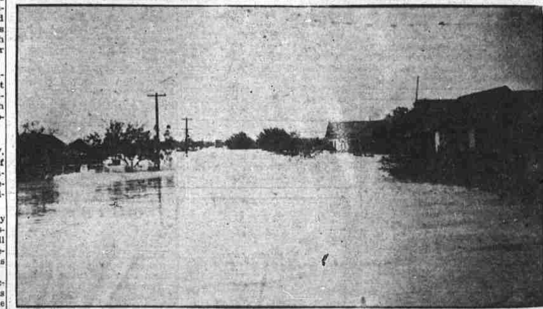
Damage ran high into the block of South Oakes street, looking south. The postoffice building is just out of the picture on the right. The picture was taken from the Cactus hotel corner. Lower view—looking down a residential street. Five homes were damaged as well as buildings in the business district. Other San Angelo flood pictures on Page 7.
