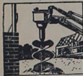
Makes holes for building foundations.
