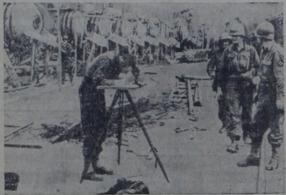
American engineers are shown surveying a 700-foot steel and concrete unfinished ramp in Normandy, which is believed to have been planned for use by the Germans as a launching site for rocket bombs. Assembly line of concrete mixers abandoned by the Nazis is in the background. Not enough and too late was the story of this Nazi effort.
