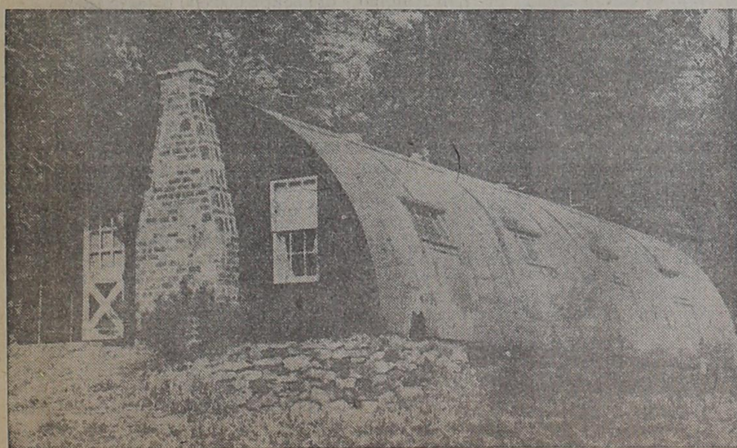
QUONSET MODEL —With government officials planning to use Quonset huts to relieve housing shortage, a Mansfield, Ohio, designer shows the attractive, as well as practical, uses of the converted model. Living room with large fireplace and shuttered windows are included. The housing shortage is one of the most acute problems in America today. A shortage had developed even before World War II. Experts say there is a demand now for 16 million additional dwelling units.
