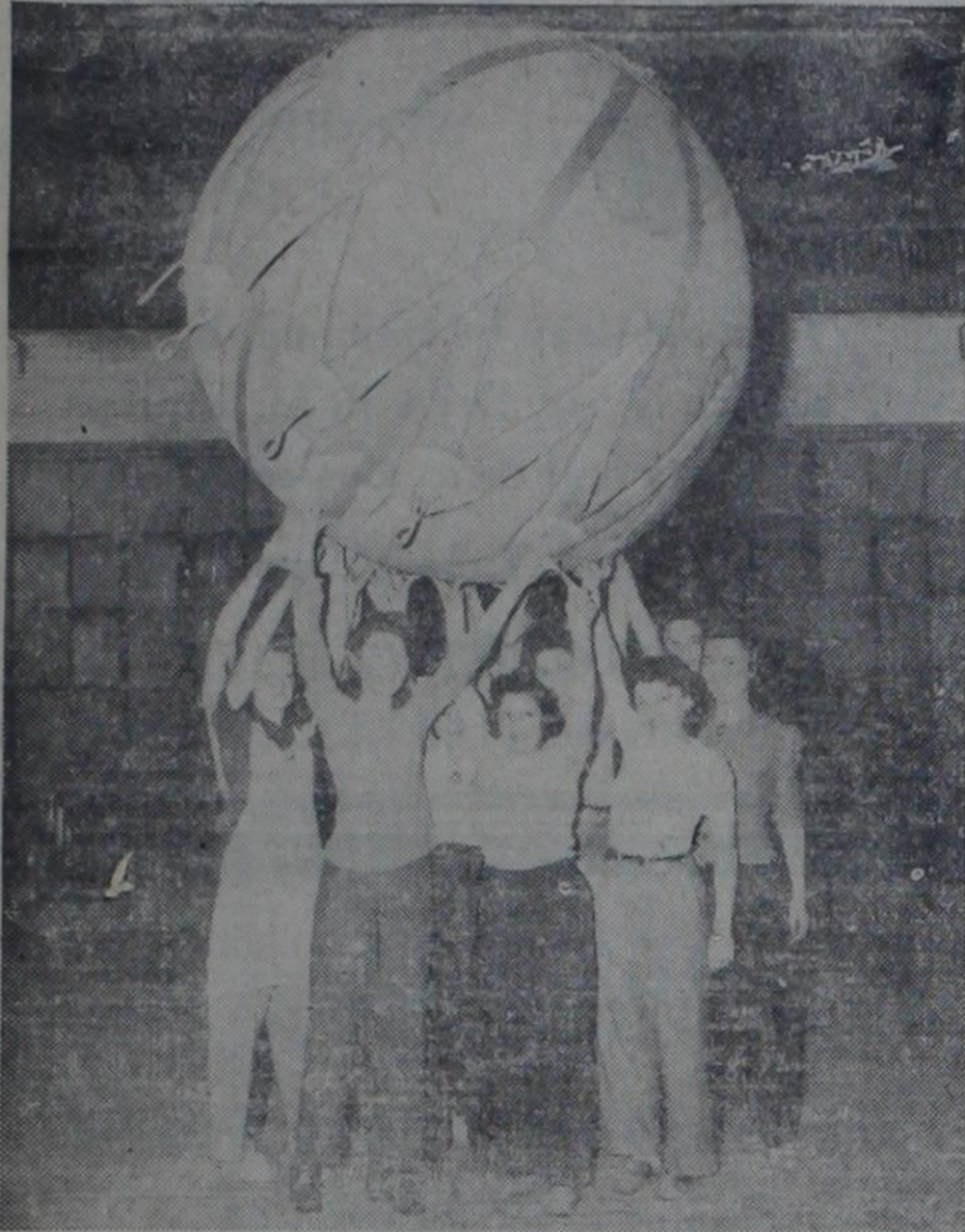
Navy planes shot down over the ocean, may be raised to fly and fight again under a plan worked out by Navy engineers. Each balloon will lift three tons and as many as five or six of them may be attached to the heavier type planes. The balloon pictured above will lift five times the weight of the girls shown holding it up.
