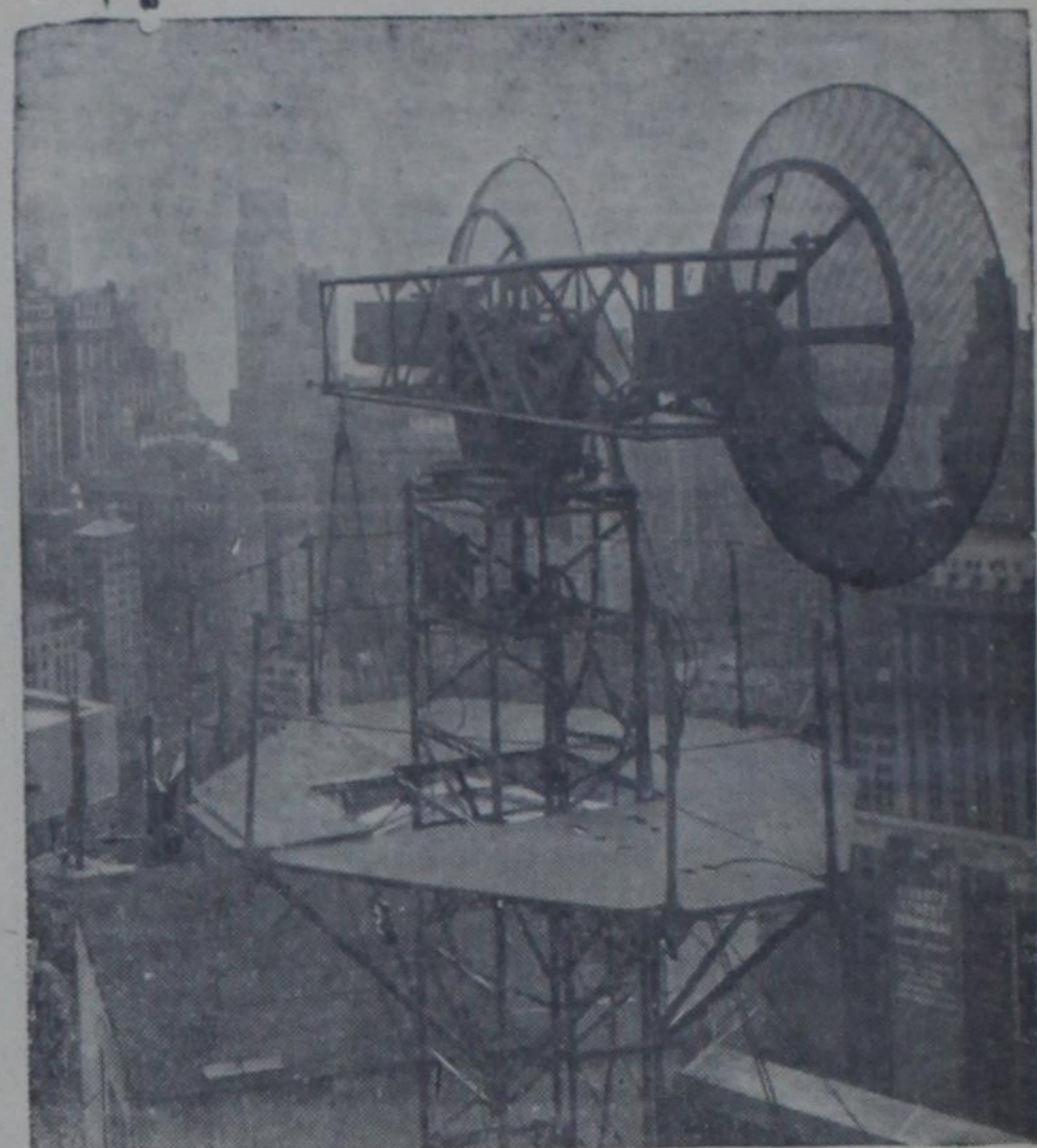
Shown atop the New York telephone building are the antennas used during demonstration of a secret army radar microwave relay system. The demonstration, conducted by Bell telephone laboratories, included a two-way voice transmission carried out successfully over links totaling 1,400 miles. It was announced as entirely practical and successful.
