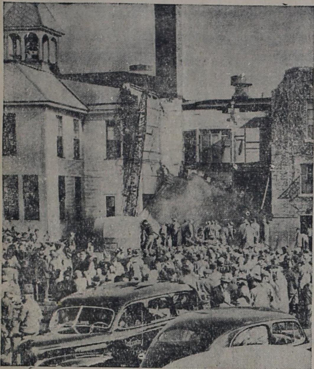
BLAST WRECKS SCHOOL . . . Crowds of anxious parents and volunteer rescue workers gathered quickly at the Baroda consolidated school at Baroda, Mich., following a boiler explosion in the basement of the school which killed one child and injured at least 16 others. When reports were first received at Chicago rescue planes with medical supplies were rushed to the scene.
