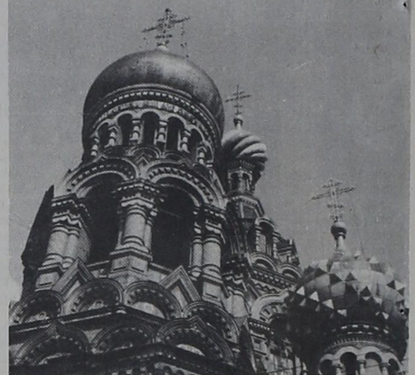
RUSSIAN CHURCH -- During their visit to Leningrad, Russia, Terri and her mother viewed the Church of the Fallen Blood. Terri reported that the church has been abandoned and windows are broken. The group did not go inside the church.
