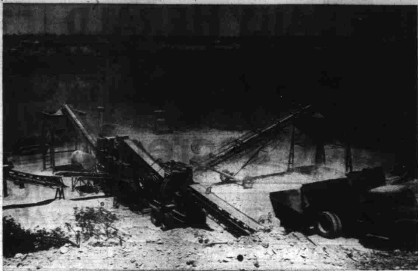
McMahon's New Crushing Plant
