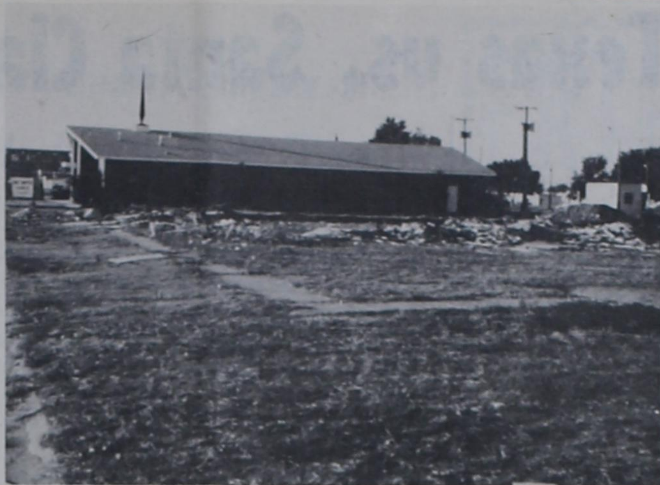
Baptist Church of Texico. On the right can be seen the new modern brick church which was built immediately south of the old building. The space formerly occupied by the old
