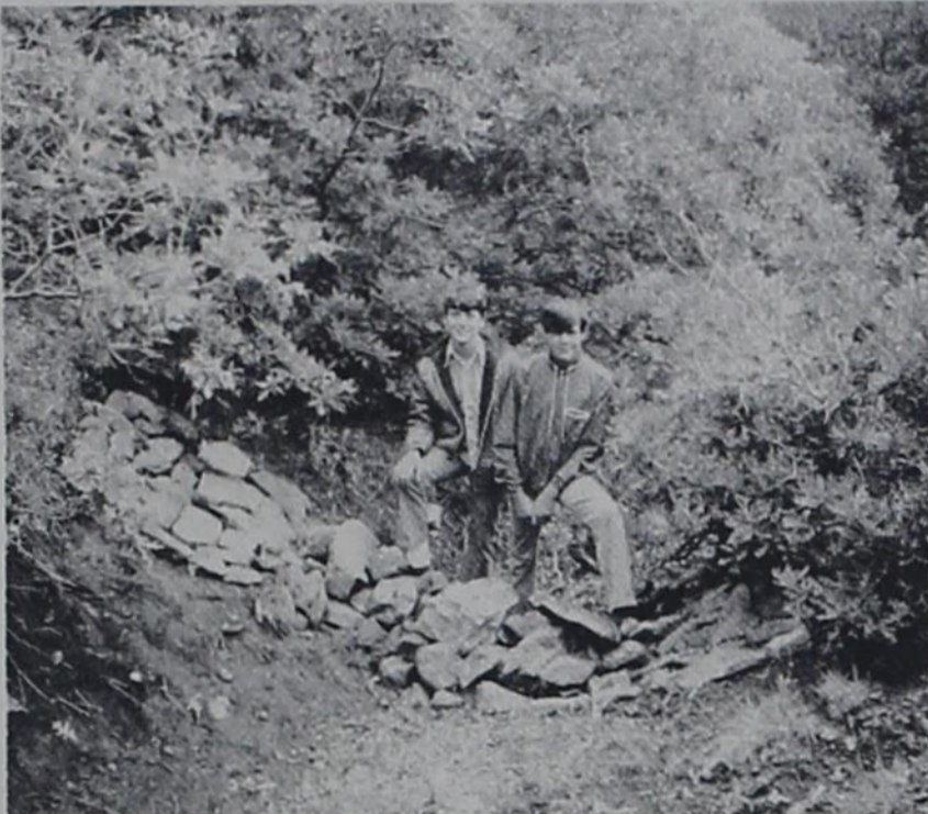
CONSERVATION PROJECT -- Troop 200 leaders Randy Stovall and Donnie Garner constructed this "check-dam" in the Cibola National Forest during the troop's July 24-26 outing there. This project was applied to advancement for Star Scout rank, and was designed to slow water flow during heavy rainstorms which hit the area each year.
