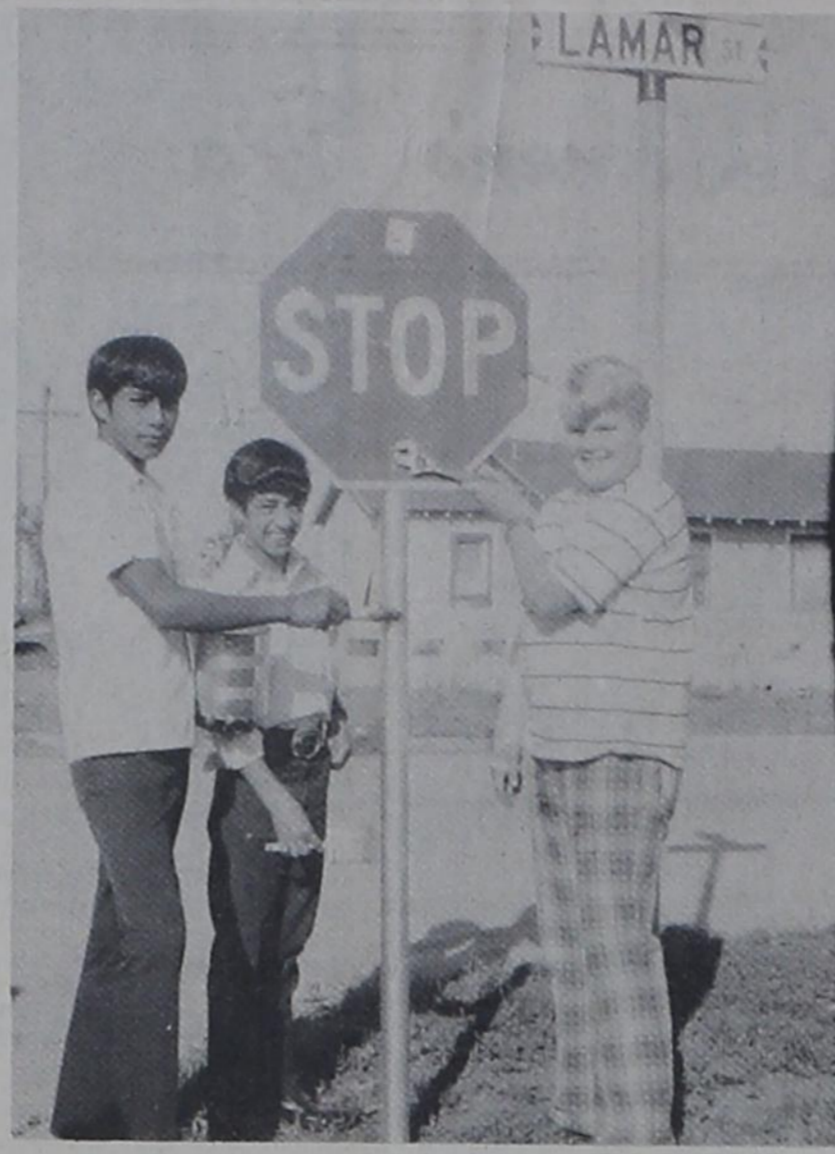
TEXICO FFA PROJECT -- The City of Texico received a face-lifting last week when Texico Future Farmers of America put up approximately 30 new stop signs on city streets. Jimmy Ortiz, left, Albert Galvan, center, and Roger Pace, right, are putting the finishing touches on the last sign. The chapter dug post holes, put the signs up and painted the posts for the signs which the city purchased. The project was a community service project. Any time there is a project with which the FFA boys could help, Eddie West, sponsor, would like to know.
