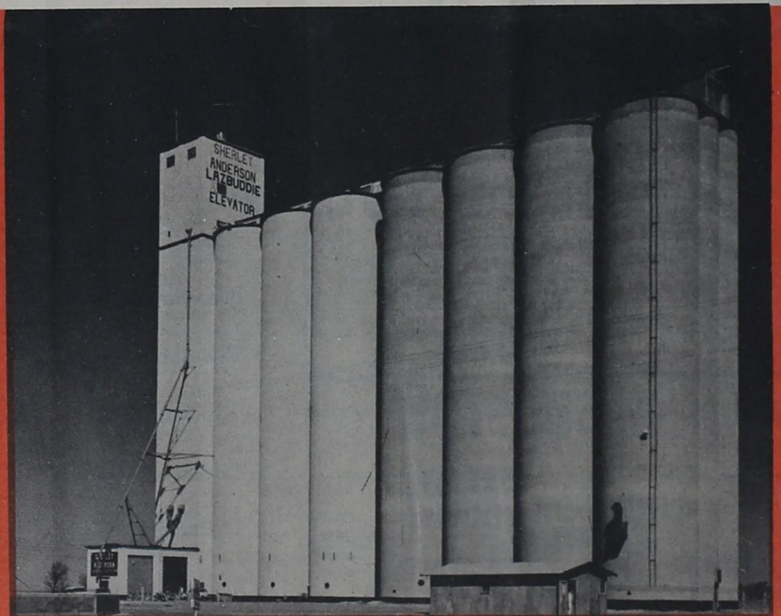
Sherley - Anderson LAZBUDDIE ELEVATOR
