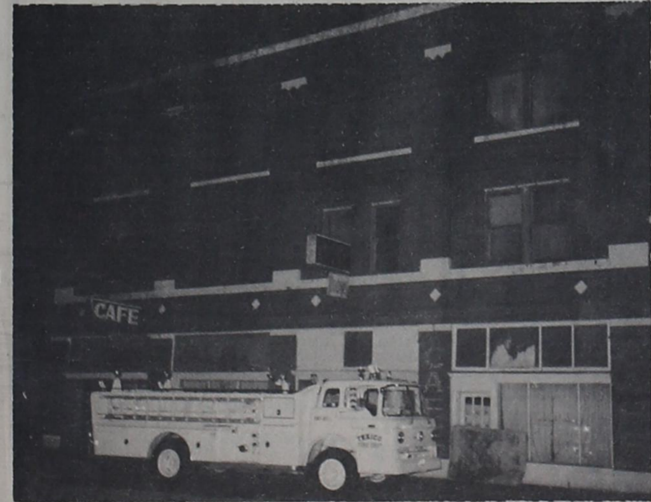
TEXICO HOTEL BLAZE -- A fire erupted in the ceiling and floor between the second and third floors of the Texico Hotel early Monday morning. Vehicles from the Texico Fire Department answered the alarm at 5:25 a.m. The firemen contained the fire almost three hours later. Smoke can be seen coming from the second window from the left on the third floor. Heavy damage occurred on the third floor and two rooms on the second floor received heavy smoke and fire damage, according to Lewis Cooper, Texico fire chief. There was a single occupant in the hotel at the time, but his room was not the one in which the fire started. Against the building to the right of the fire truck is a mattress which was removed from one of the burning rooms.
