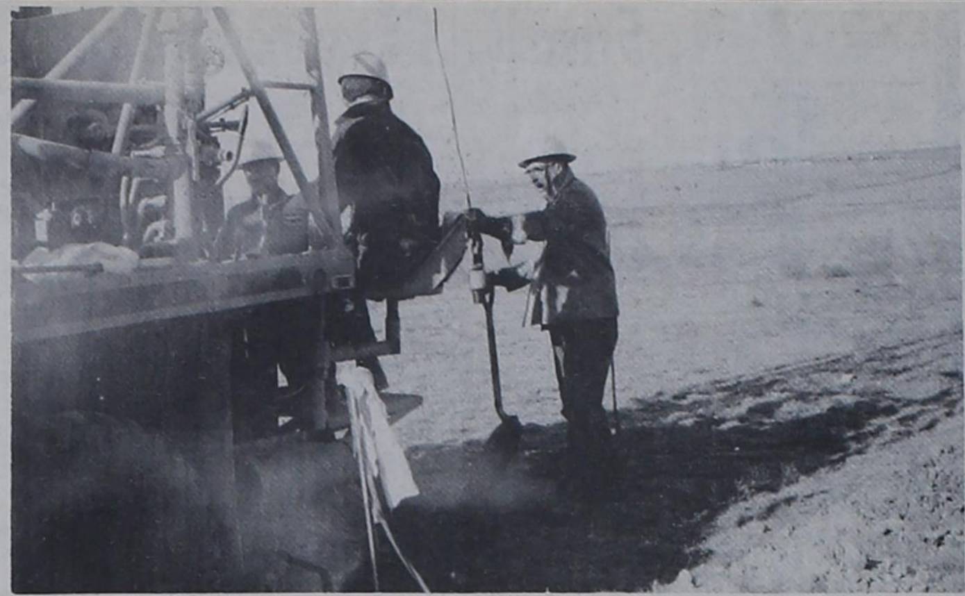
WATERSHED PROJECT -- A Soil Conservation Service Core Drilling crew is pictured working in the Running Water Draw Watershed on the R. J. Sanderson ranch near Lazbuddie. Two flood prevention structures are scheduled to be built in Farmer County. One structure is to be located about one mile north of Bovina and the other about five and one half miles northeast of Lazbuddie.
