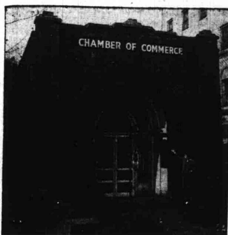
HOUSE OF COAL—The Chamber of Commerce building at Williamson, W. Va., is built of solid bituminous coal. Miners and operators joined in raising the structure in 1933.
