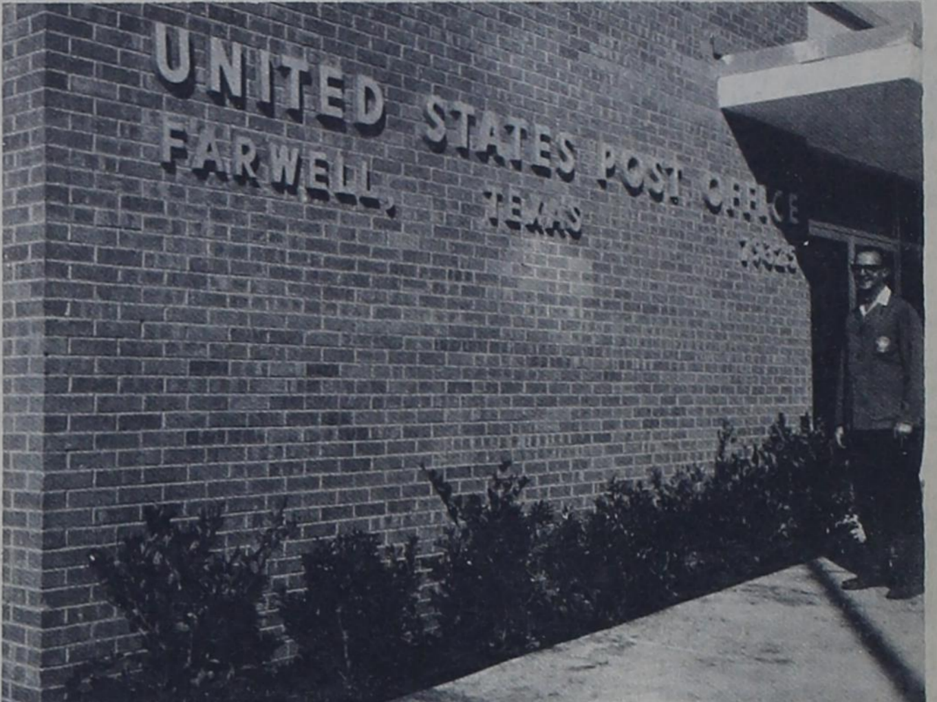
ALMOST READY -- Postmaster Jim Bob Smart looks with pride at the newly-constructed post office building into which local postal employees hope to be moved by end of the week. The building was accepted by postal officials on Monday.
