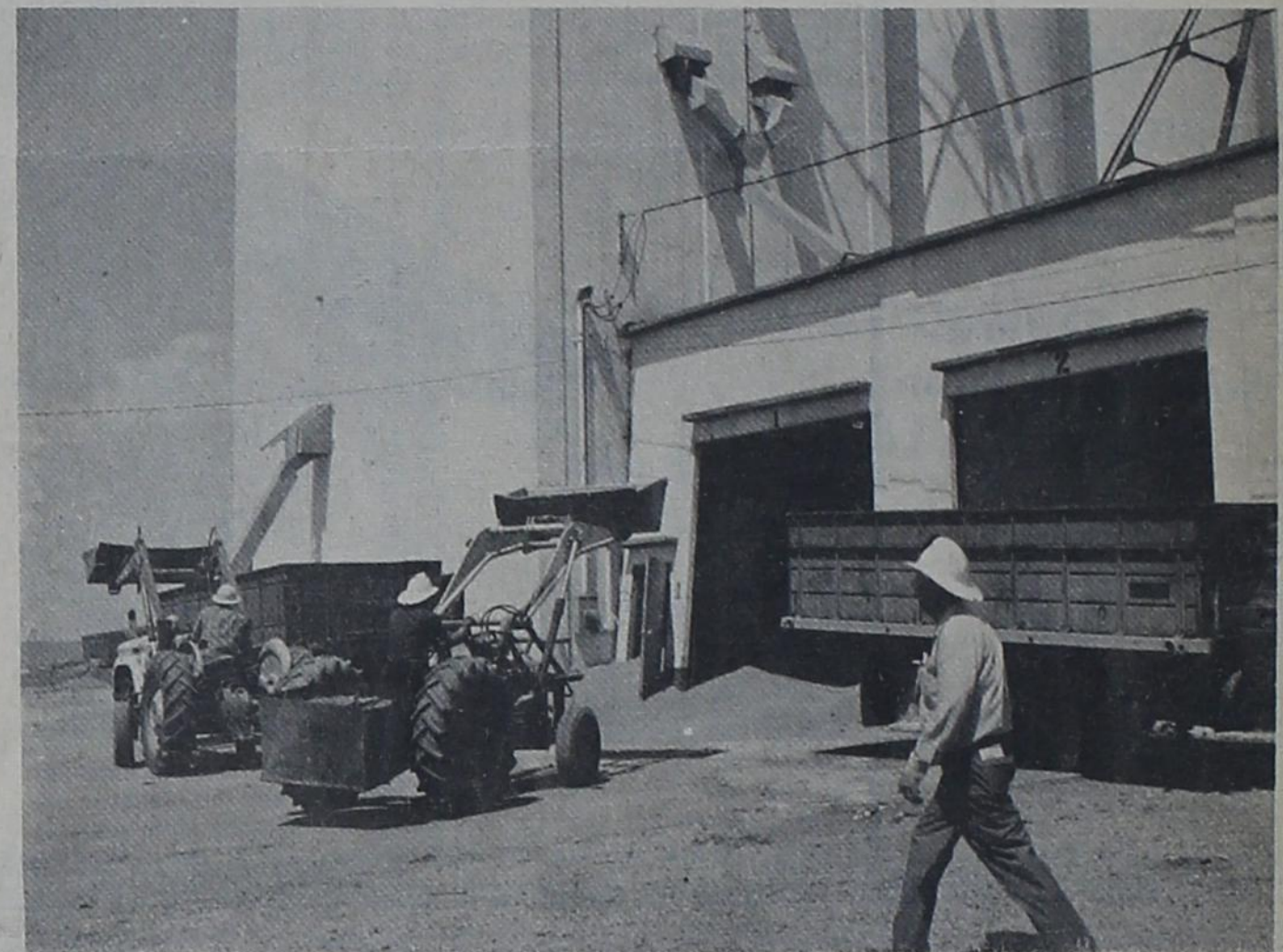
CARRY AWAY DEBRIS -- Volunteer workers carry away grain and debris from the wreckage of the elevator in which the body of Cloys Stanberry was imprisoned. About 50 workers spent five hours in the rescue attempt. Two other workers were injured in the blast.
