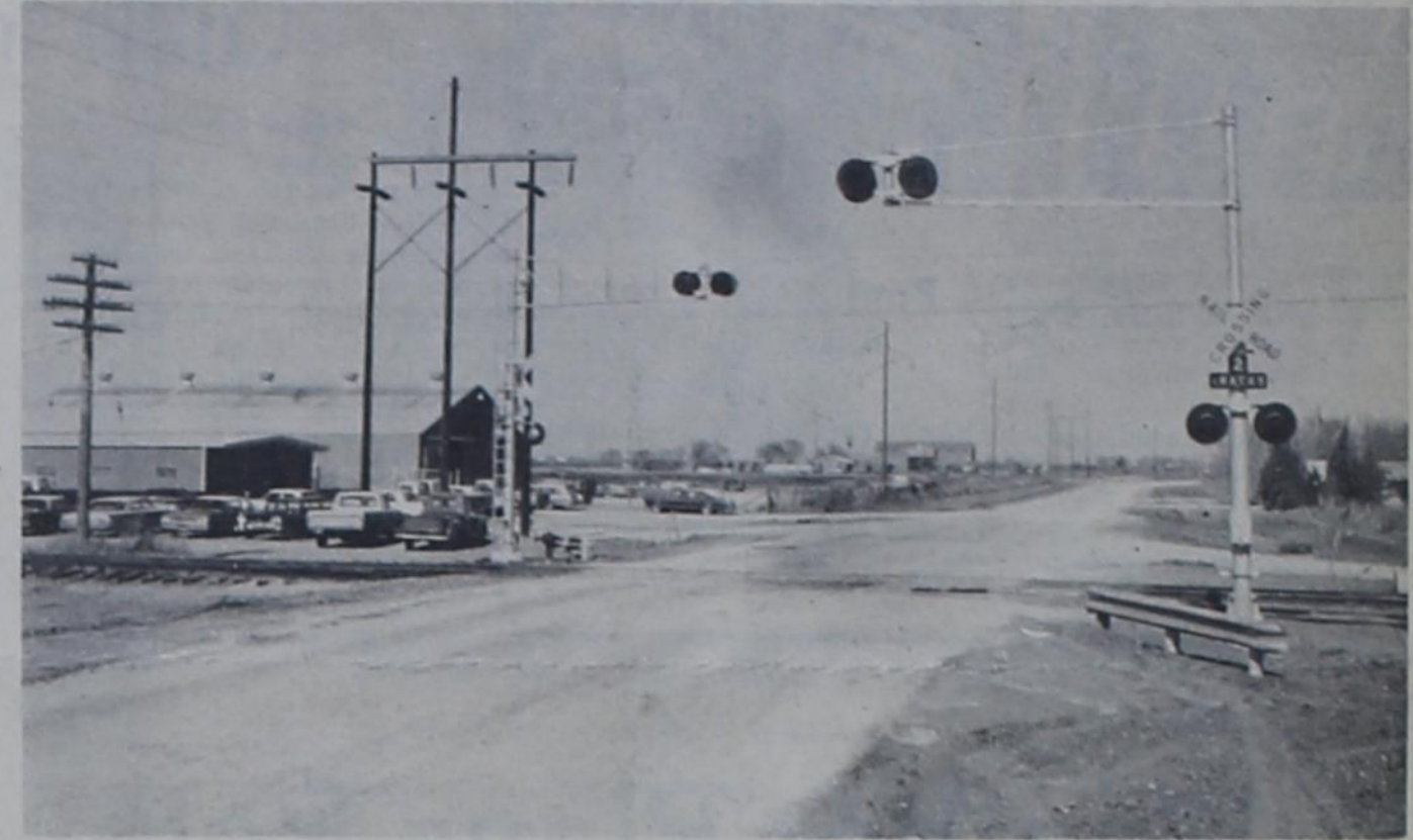
New signals have been installed at the railroad crossing on the road which links Highway 70-84 with Highway 60 near Gifford-Hill-Western and Sherley-Anderson-Pittman elevator in east Farwell.
