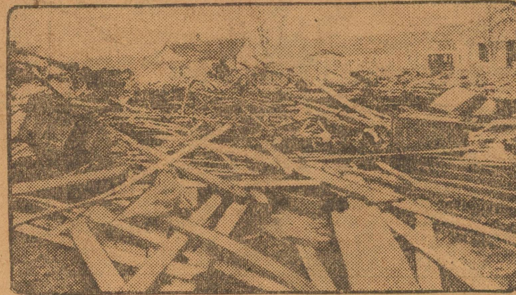
The picture above shows the home of W. E. Smith, of Fairfax, Okla., before it was wrecked by an explosion that killed Smith, his wealthy Indian wife and a white servant girl. The picture below shows the wrecked home. A federal grand jury is investigating charges that the explosion was part of a murder ring's plot to gain the wealth of many rich Osage Indians.
