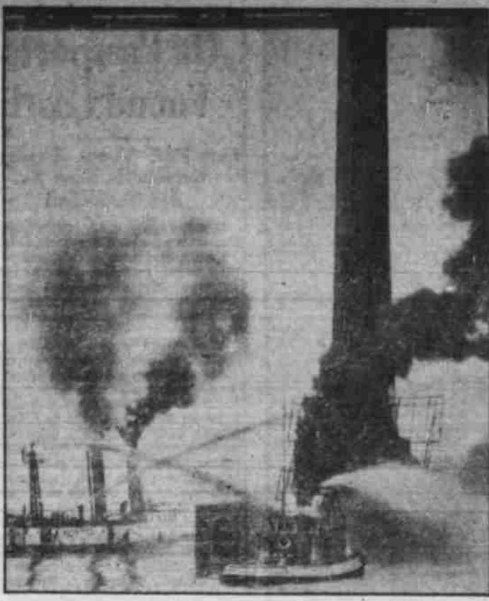
Two fireboats are shown as they played water on the blazing creosote piling at a pier on the $75,000,000 bridge being built from San Francisco to Oakland. Several workmen were forced to leap into the bay for their lives. Others were rescued by an army launch. (Associated Press Photo)
