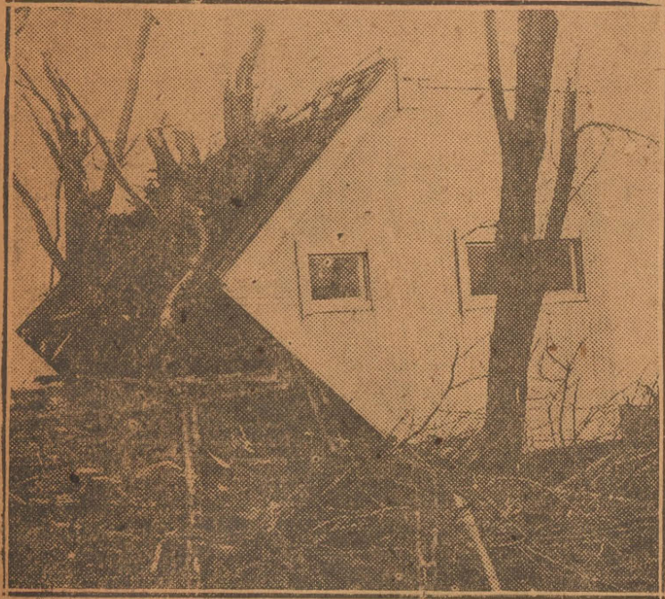
The storm played strange pranks. Here is a house turned on its side and lodged between two trees on Main street of Griffin. The glass windows were not broken.
