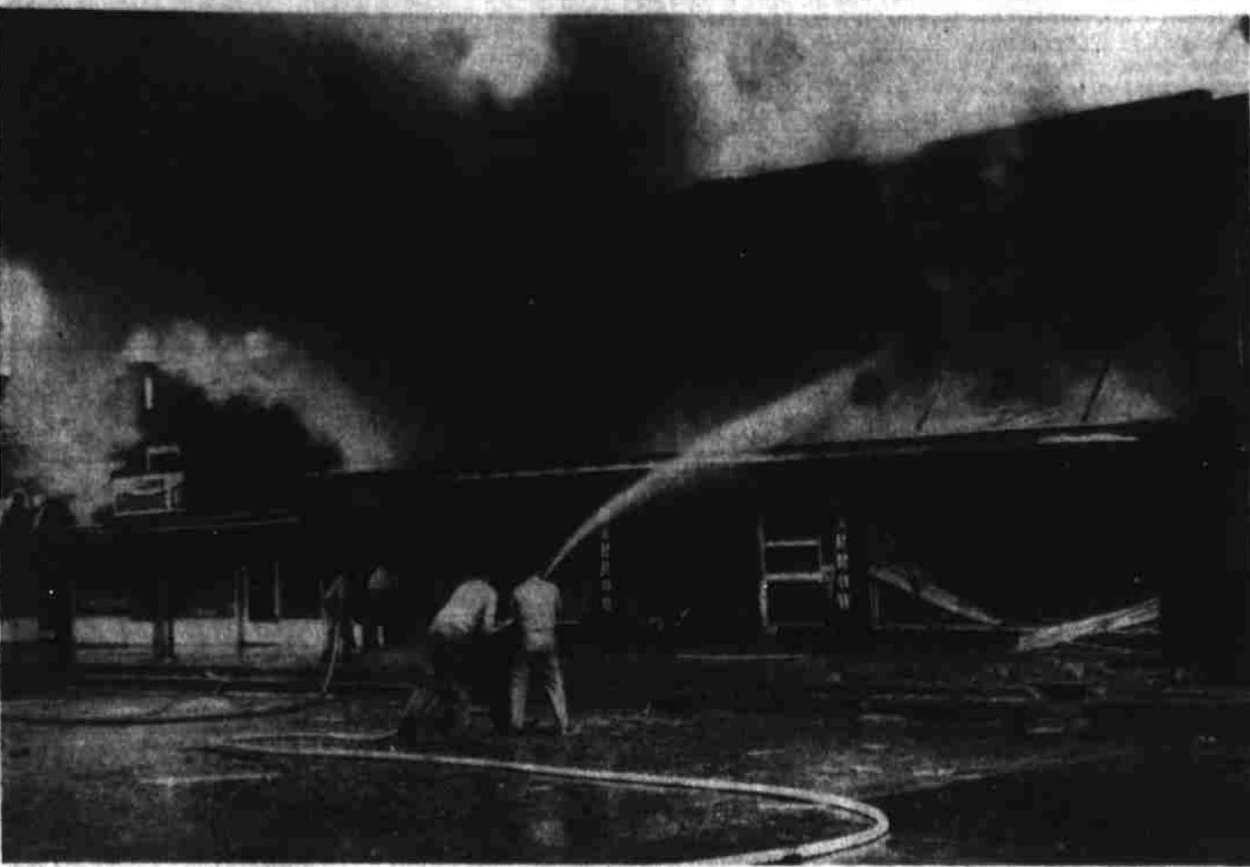
BLAZE AFTER BLAST — Firemen throw water into the blazing interior of the Barrow-Douglass Furniture company, 205 Rannels, as fire followed an explosion late Friday evening. It took determined work on the part of the firemen to save adjoining buildings. Three were injured in the explosion, and the resulting fire is rated the city's worst since the compress fire in 1938. Although definite estimates were not immediately available, preliminary surveys indicated the loss would be around $100,000. — See additional fire pictures on Page 5. (Culver Photo).
