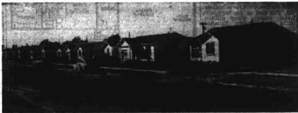
Taken in the 1300 block of Martha, the above picture shows another grouping of homes erected by Big Spring Lumber.
