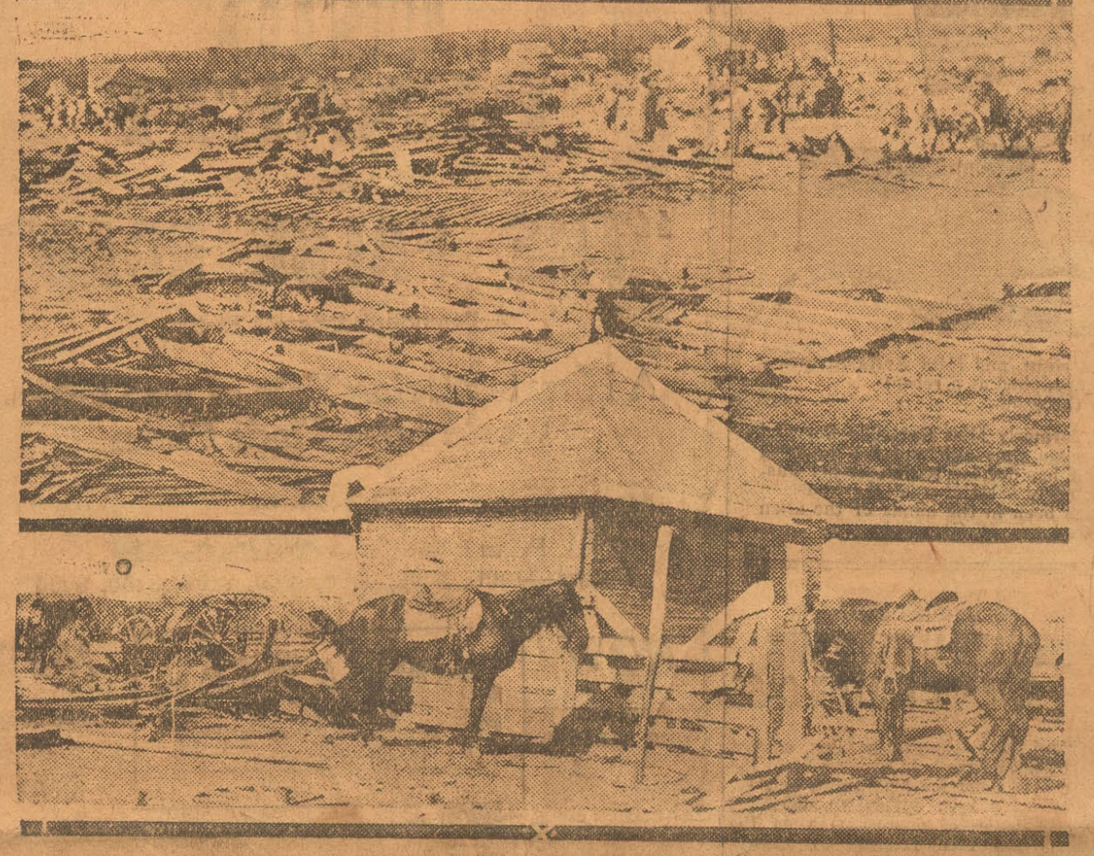
All that is left of the heart of the town of Peggs (above) and the "city jail," the only building in Peggs left unscarred by the storm.
