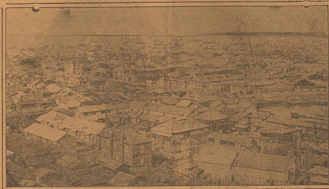
Here is a panoramic view of Yokohama, Japan, where tens of thousands perished in earthquake, fire and flood.
