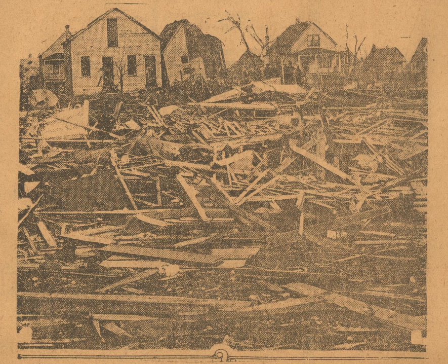
A Scene at Seventy-first Avenue and Dakin Street, Chicago. At least twenty-nine persons were killed in Chicago, and hundreds were injured when a tornado struck the outskirts of that city last Sunday afternoon. The photo gives a glimpse of the devastated area.
