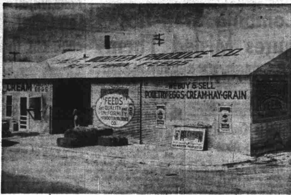
NEW PLANT—Harvey P. Wooten has erected and moved into a new plant at 504 E. Second street, where he offers the same complete lines of Red Chain feeds, together with hay and other feed needs for any kind of fowl or animal. Besides this, Wooten's new building is especially designed for his cream, butter and egg purchases and for processing poultry. The plant is conveniently located on a wide, paved street. (Jack M. Haynes Photo.)
