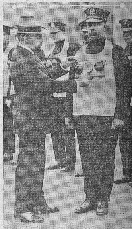
LIGHTS ON NIGHT POLICEMEN —A new signal device to be used by the night traffic policemen of New York City, was demonstrated by Department Commissioner Dr. John A. Harriss, who originated the device. It consists of three lights—red, orange and green, and is suspended upon the chest of the officer, on top of a sort of apron-like jacket of white.
