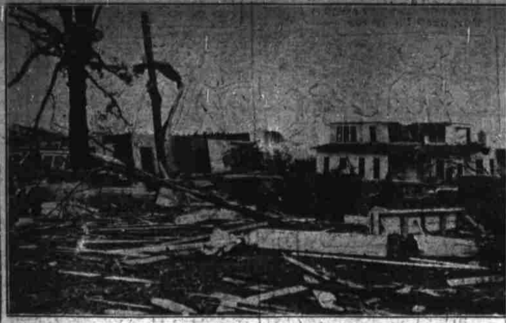
This picture shows damage caused in a residential section of Minden, La., by May day tornadoes which tore through northern Louisiana and southern Arkansas, killing scores and making hundreds homeless. (Associated Press Photo)
