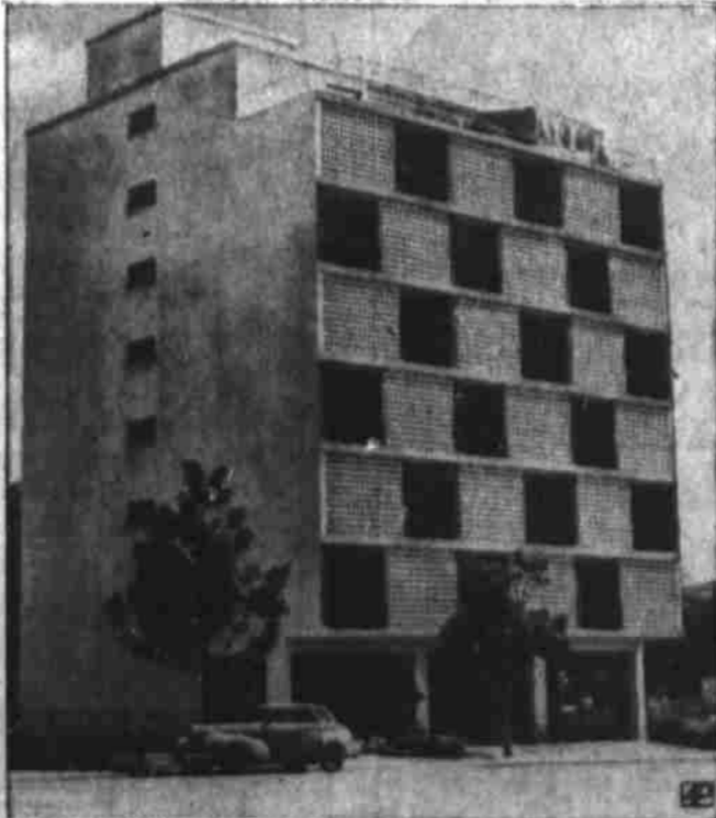
MODERN DESIGN — Beehive brick design on the balconies of apartment house development in Caracas, Venezuela, creates a natural air flow and protection from the tropical sun.
