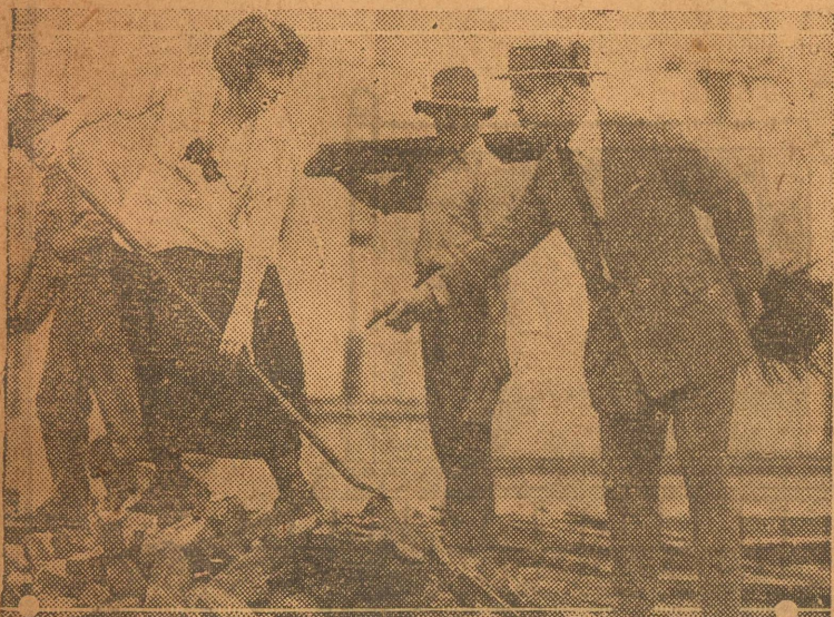
MRS. CARROLL STARTS THEATRE —Using a crowbar, Mrs. Earl Carroll began work recently on the site for the theatre Earl Carroll, song writer and producer, is to build in New York. Work will be pushed on e, which the owner expects to open about Christmas. The Mrs. Carroll at work, while Mr. Carroll directs.
