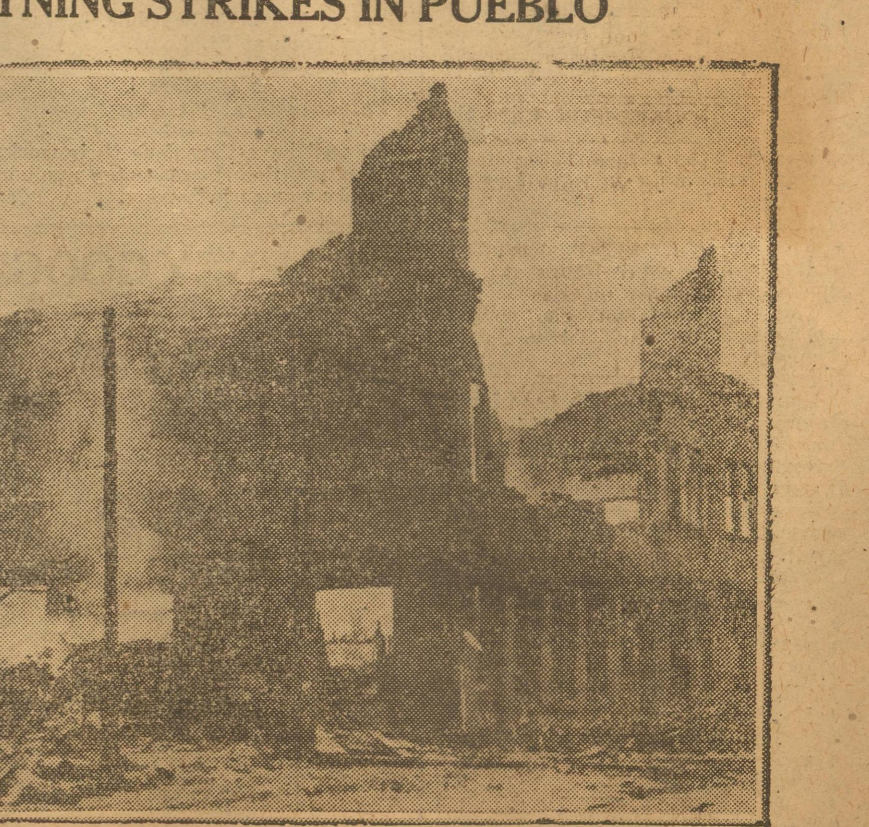
This photograph shows Foley's lumber yard in Pueblo after it was struck by lightning during the flood. Numerous fires were caused throughout the city as the burning lumber from the yard was carried about on the crest of the waters.
