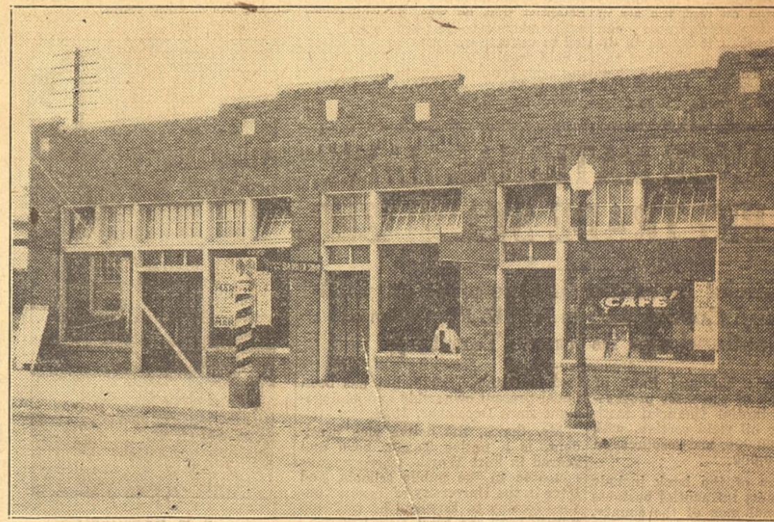
THE HARNESS BUILDING RECENTLY CONSTRUCTED BY WHITEHALL
