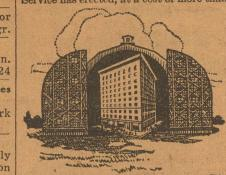
\$2,000,000, a large airship hangar. The huge structure could contain a 10-story office building with a 50-foot tower on the roof. The hangar, which is built of steel, concrete, and glass, is 825 feet long and 225 feet high. At the end are large steel doors opened and closed by electric motors that travel on railroad rails.
