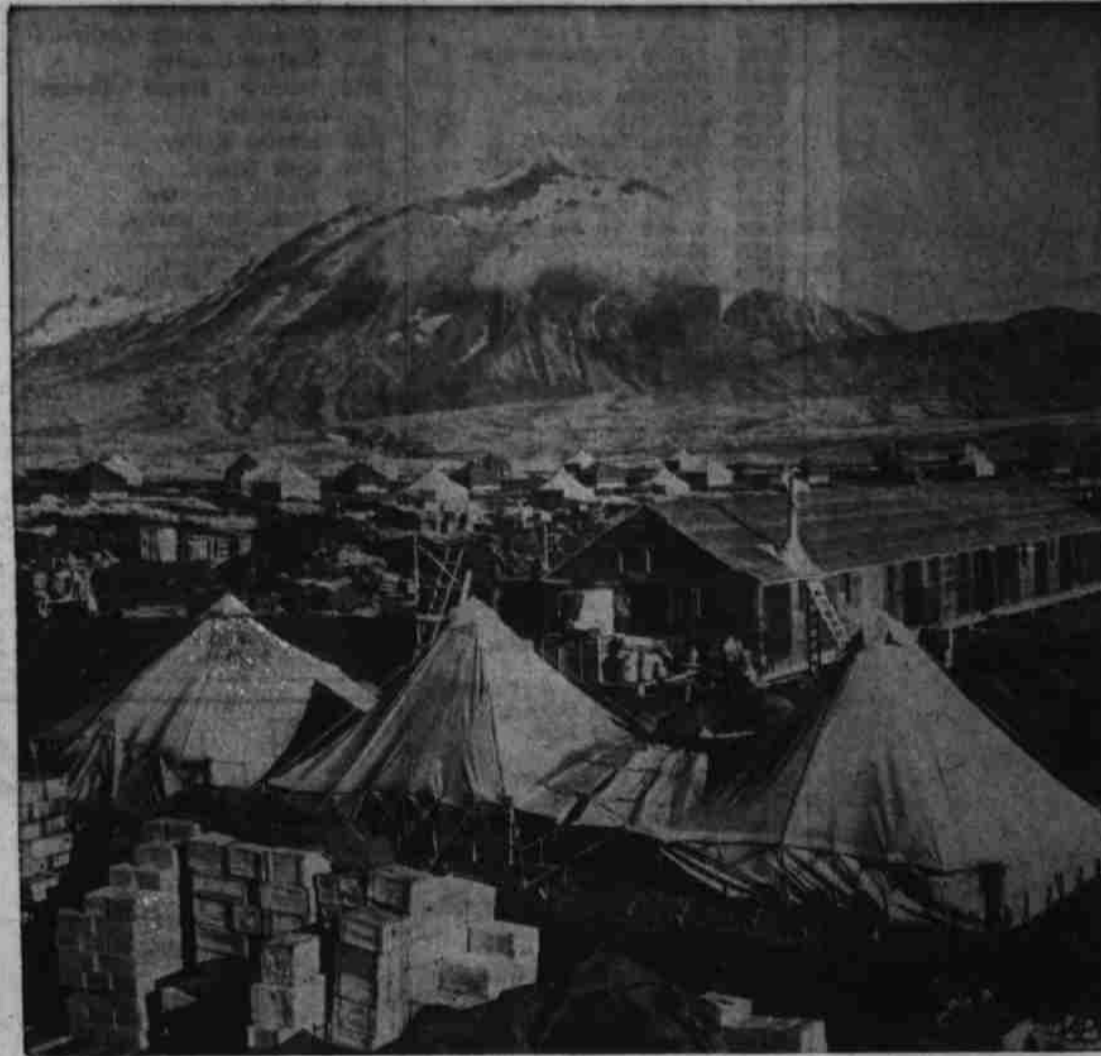
TENT CITY RISES ON ATTU —With a snowcapped mountain in the background, a tent city, forerunner of a permanent base now under construction, houses U. S. forces on Attu Island.
