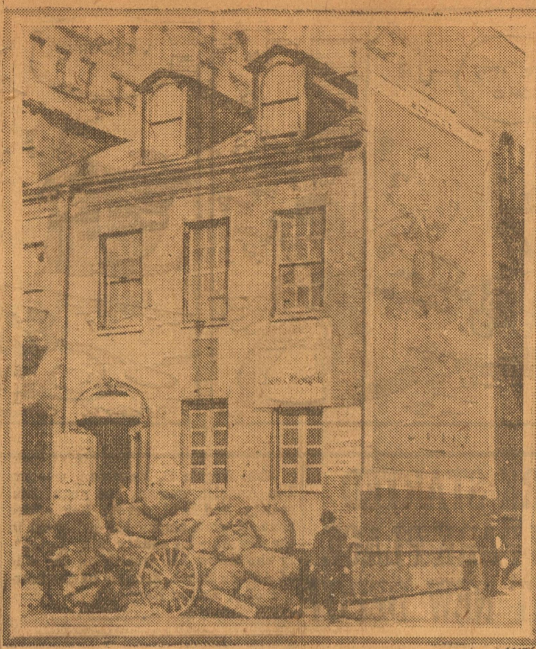
The old house at No. 63 Prince street, New York, where James Monroe, fifth president of the United States and author of the famous Monroe doctrine, died July 4, 1831, is to be torn down to make way for a modern twelve-story factory.
