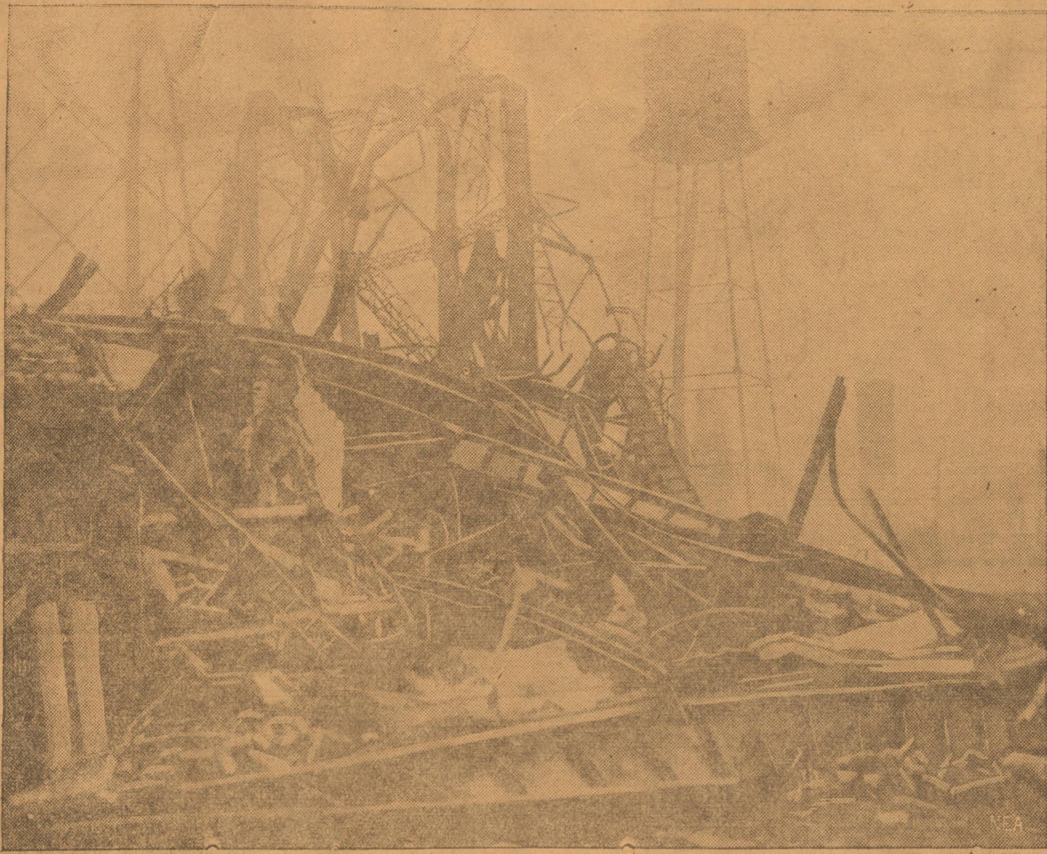
This graphic picture shows the wreckage of the Reedsdale plant of the Equitable Gas company, at Pittsburgh, after a 5,000,000-cubic foot gas tank exploded. Many people were killed and scores were injured in the blast, which rocked all of Pittsburgh.
