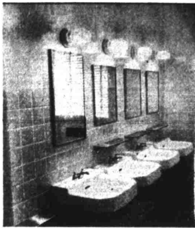
FINE FIXTURES—Typical of the fine appointments throughout the Veterans Administration hospital here is this washroom. Floors are ceramic tile, the walls glazed tile, and the lavatories, of course, of enamel ceramic with stainless steel fixtures. Mirrors are individually illuminated. (Culver Photo).
