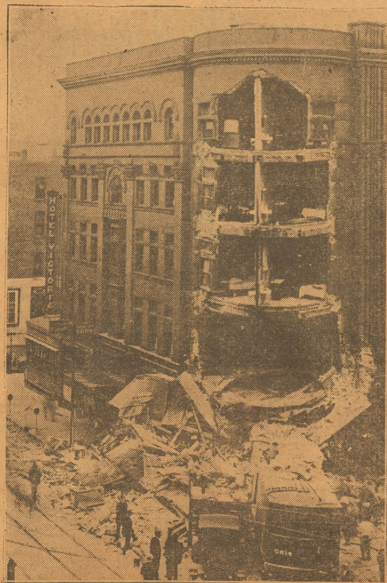
TROLLEY CAR CAUSES DRAUGHT —A three-car electric train, bound from Worcester to Springfield, Mass., jumped the track on the incline at State street and smashed into the Victoria Hotel. The impact tore away the supporting pillars and the fallen wall left open the hotel sleeping rooms on the upper floors.
