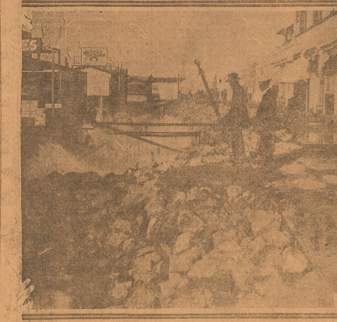
How waves washed away sea wall and emergency 'fill' at one section of the wall, leaving pier used by concessions practically unconnected with the mainland.
