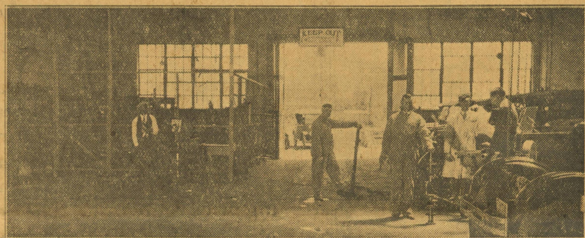
Modern shop under the direction of R. A. Arnold, service manager; and competent force of skilled mechanics to service Studebakers and Chevrolets.
