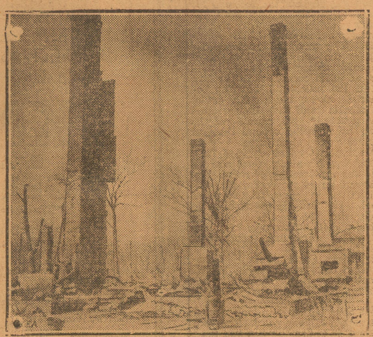
Fifteen hundred people were made homeless when a high wind swept a fire through 30 blocks at Newport, Ark., destroying 325 houses. This picture shows the ruins of the home of R. J. Hugley, who had moved in only two days before. A few months ago he lost a former home by fire.
