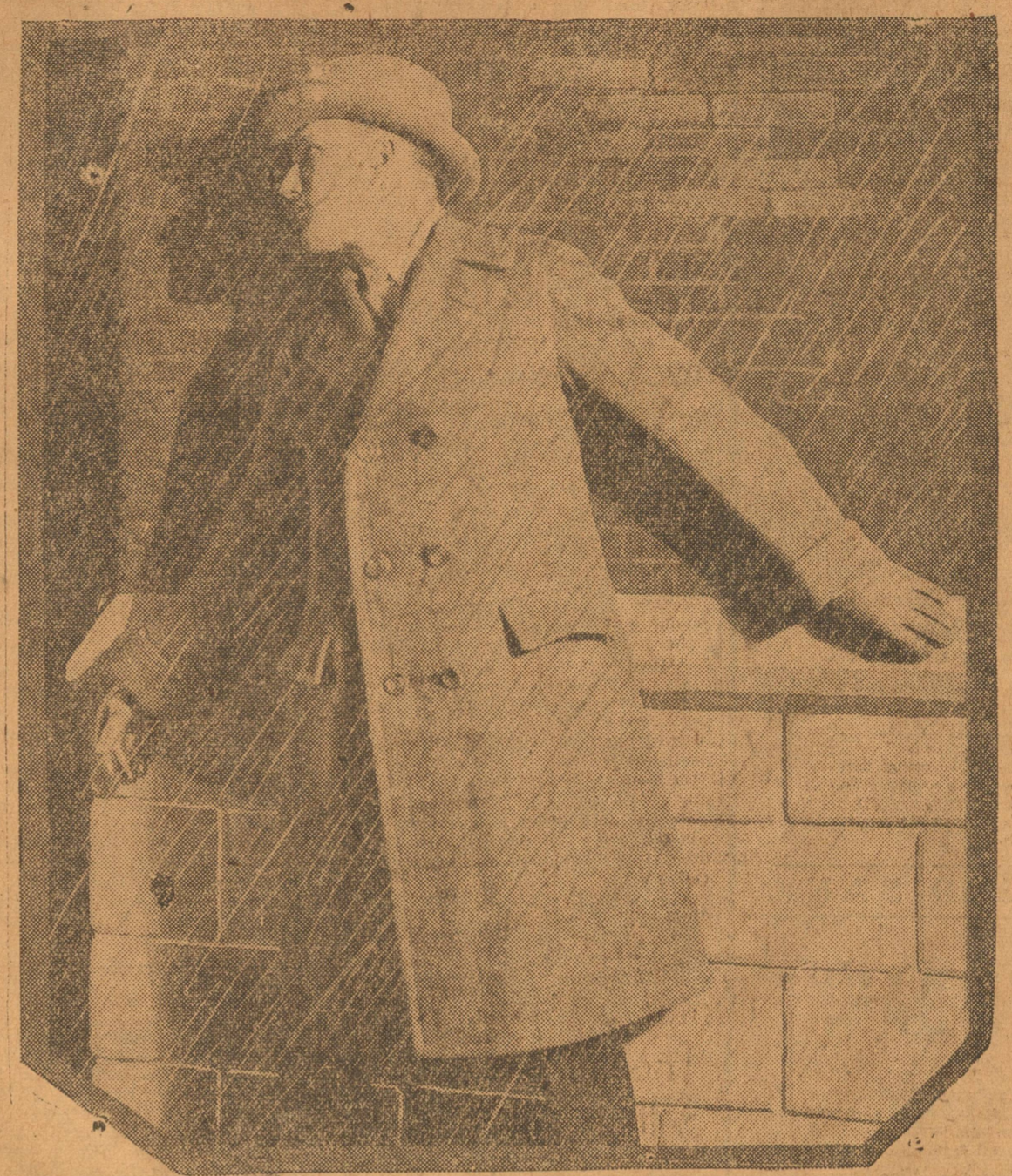
Jimmy pressed himself flat against the building and waited.
