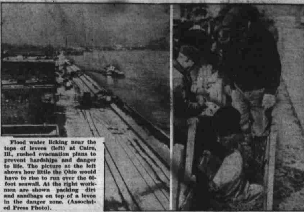
Flood water licking near the tops of levees (left) at Cairo, Ill., rushed evacuation plans to prevent hardships and danger to life. The picture at the left shows how little the Ohio would have to rise to run over the 60-foot seawall. At the right workers are shown packing dirt and sandbags on top of a levee in the danger zone. (Associated Press Photo).
