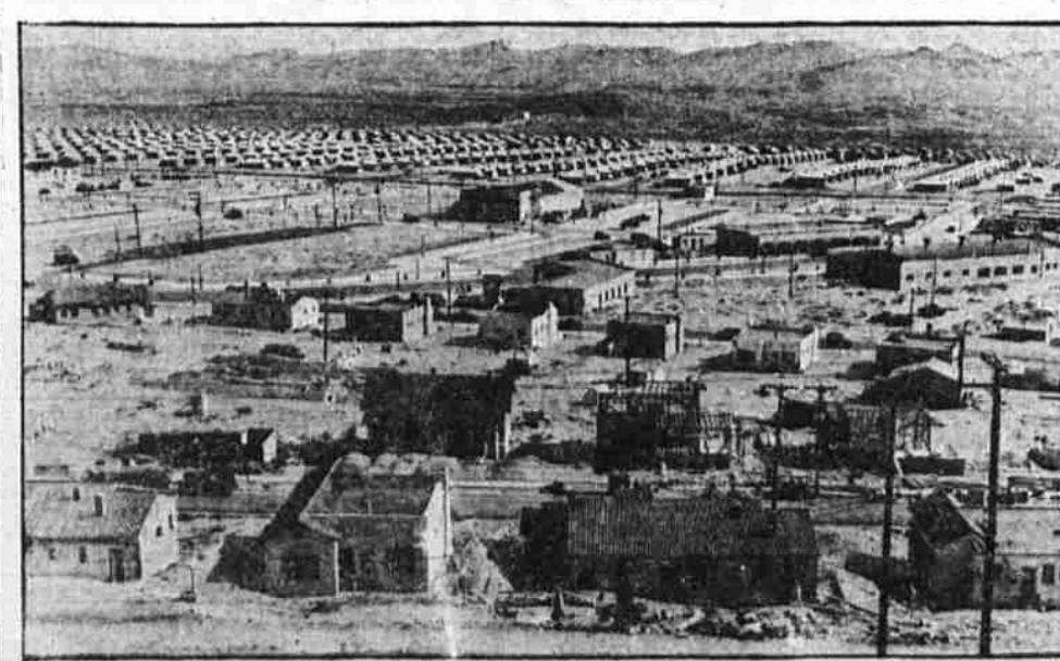
This view shows a section of Boulder City, Colo., a "model" town built about eight miles from the site of the Hoover dam to house workers employed on the project. Thirty-five hundred men and their families live there, the workmen being transported to and from their work in buses.
